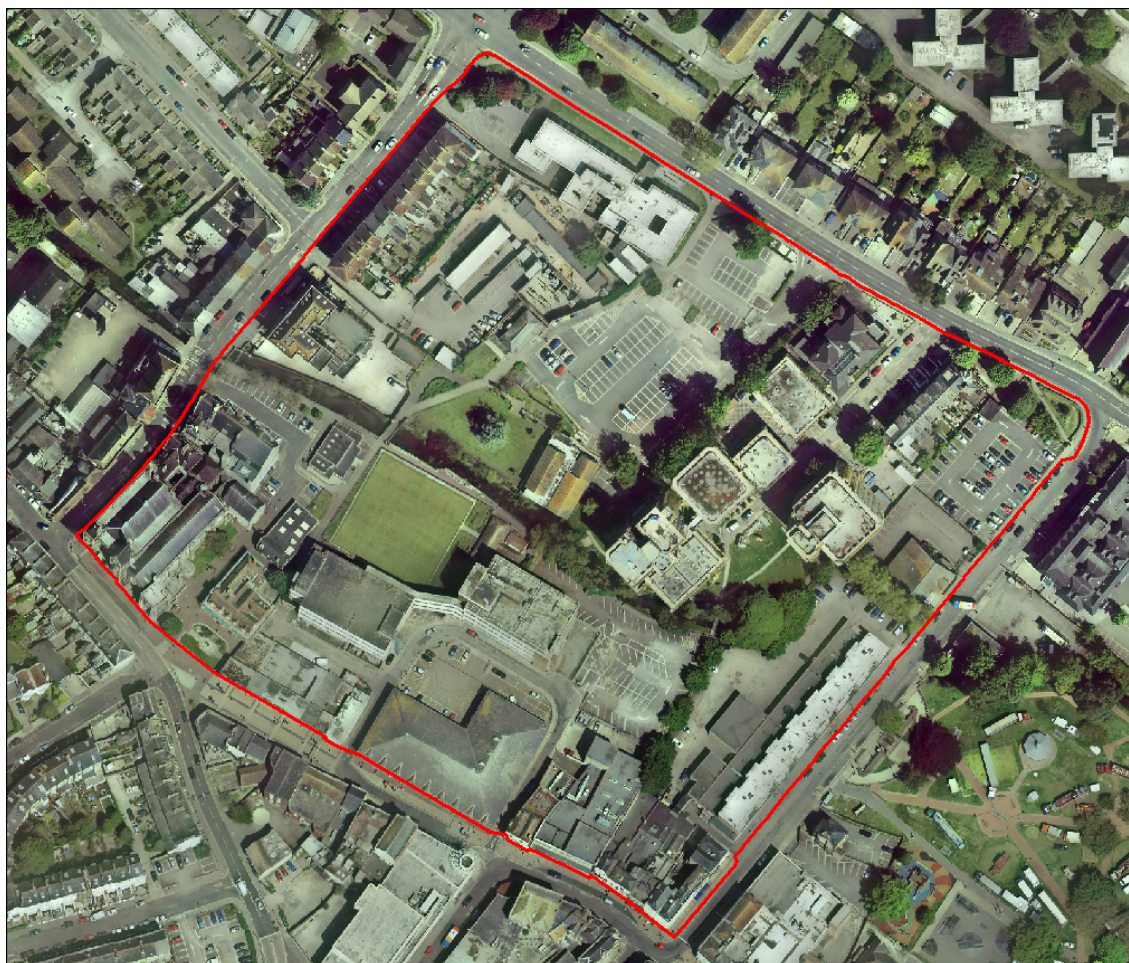
Aerial photograph of Mid Town
